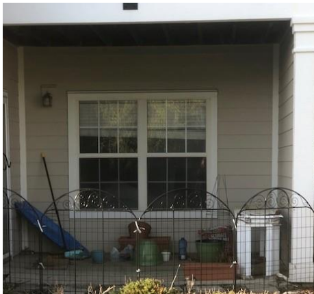
*Patio NOT in compliance with TCC Rules Regulations.
